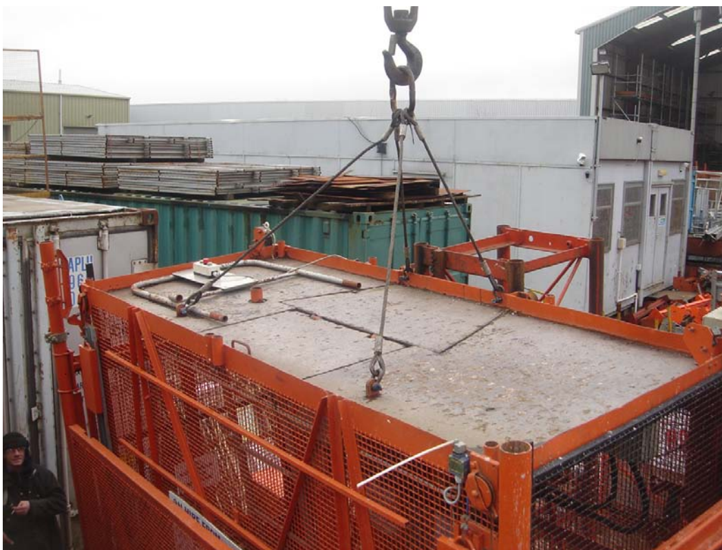
Figure 2 - Sling Master Links Attached to Lorry Loader Hook
