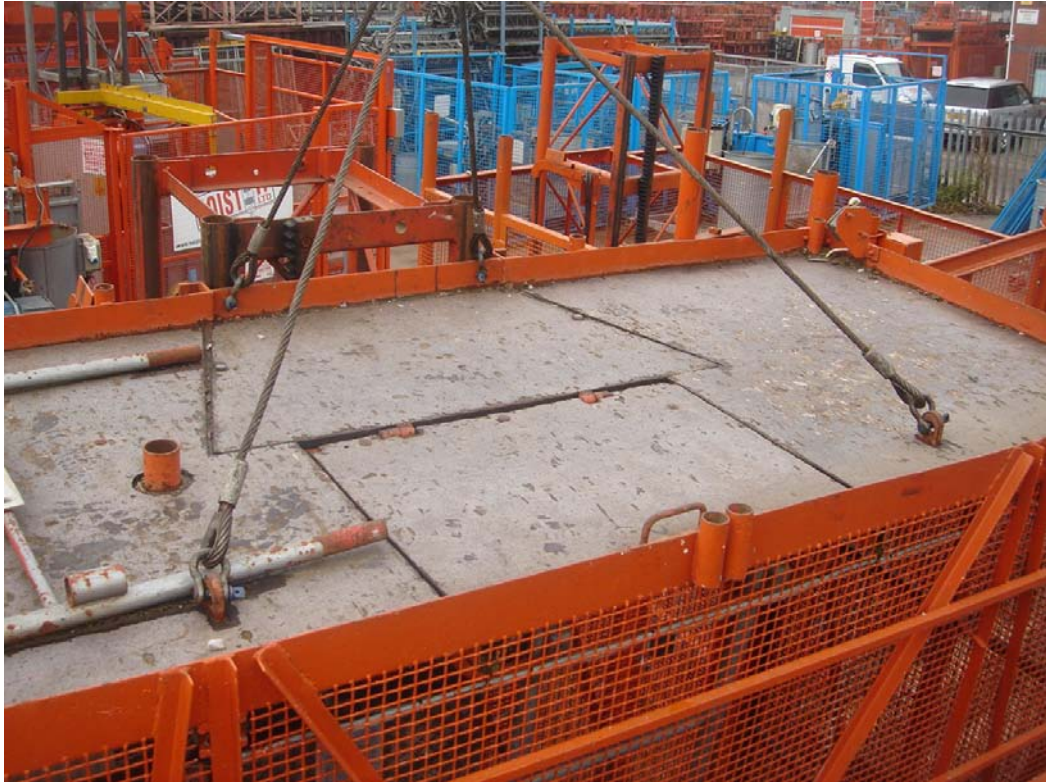
Figure 1 - Installation of Slings to Cage Lifting Points
